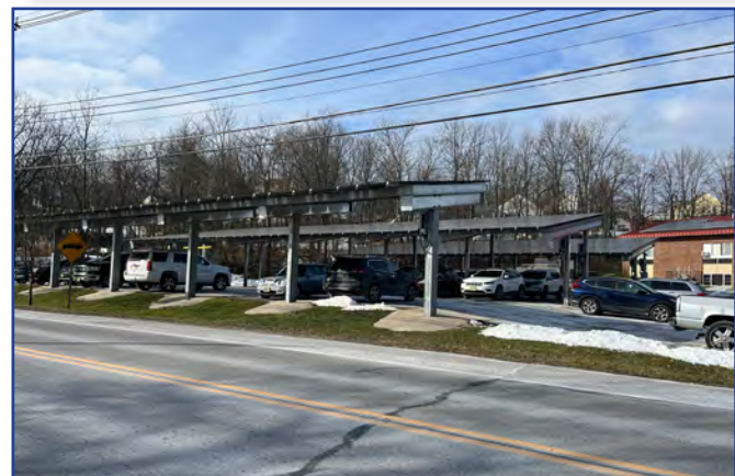
Images 77 and 78. Sussex Middle School has two parking lots that are less than ¼ mile from Main Street which could be utilized as overflow.
