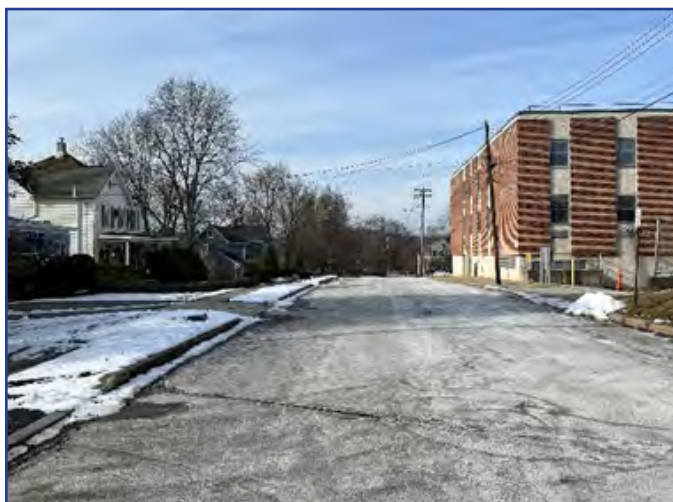
Image 110. The rear of the former Saint Clare’s Hospital on Sycamore Street in an otherwise residential neighborhood.
