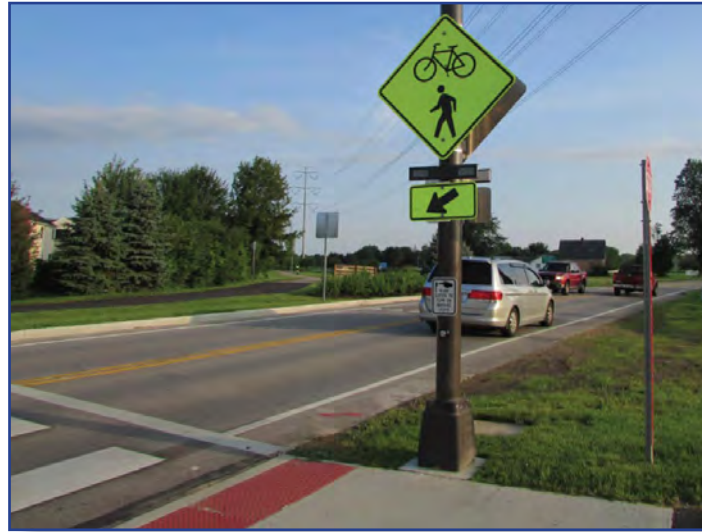
Image 85. The flashing lights of a Rectangular Rapid Flashing Beacon (RRFB) are typically activated with a pedestrian pushbutton to signal to drivers that pedestrians are waiting to cross the street.
