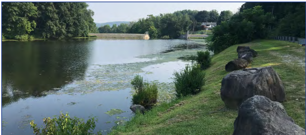
Image 67. View of dam separating Clove Lake from Clove Brook.
