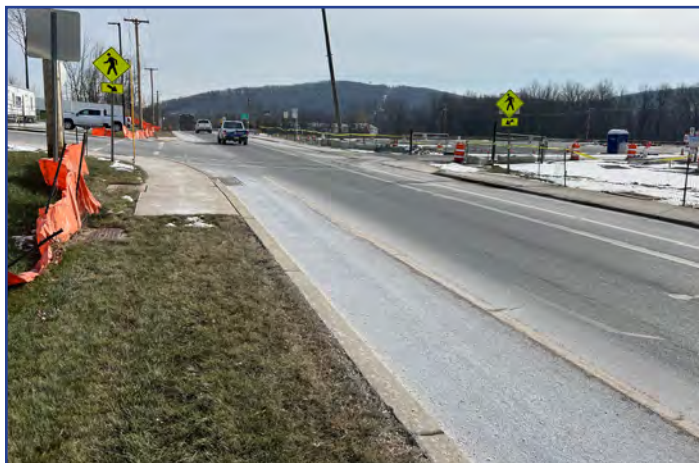
Image 84. Pedestrian infrastructure at the intersection of Walling Avenue and Wiebel Plaza across from the Shop Rite under development. Vehicle traffic rarely yields to pedestrians waiting to cross at these locations despite the “pedestrian crossing” signage.
