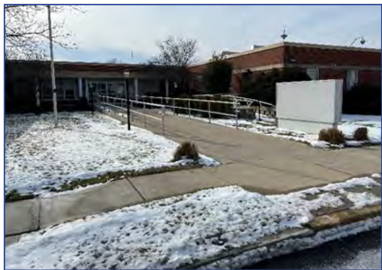
Image 109. The entrance to the former Saint Clare’s Hospital.
