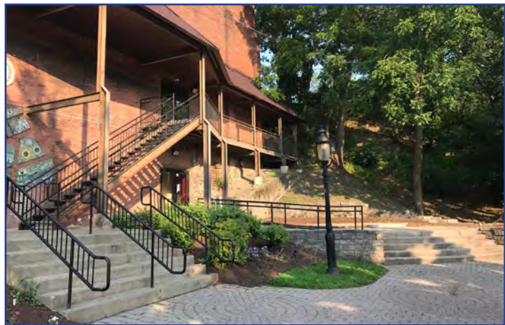
Image 61. Stairs leading to the Harrison Street Parking Lot from Deckertown Commons along the Crescent Theatre
