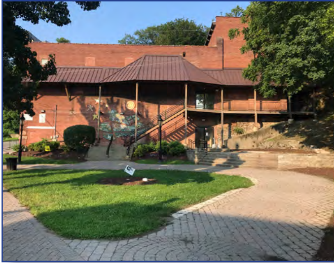
Image 42. Deckertown Commons to the south of the Crescent Theatre.
