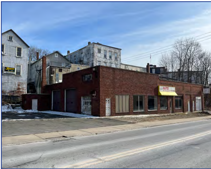
Image 13. The former Capri Auto Body building is the only remaining structure on the block of Mill Street (State Route 23) between Newton Avenue and Loomis Avenue. This building partially obstructs the view of Main Street buildings while its vacancy in a prominent location suggests to drivers that this is representative of the Main Street area as well as the Borough.
