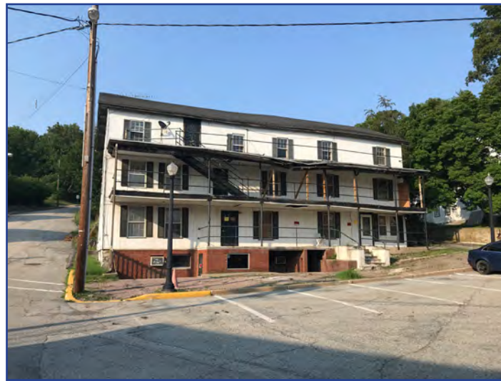
Image 98. The former Fountain Square Inn is vacant and uninhabitable in its current condition.
