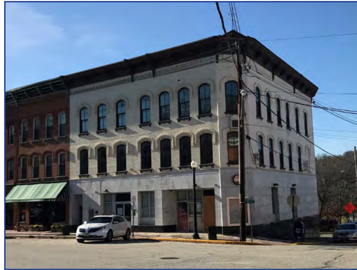
Image 99. The former Chase Bank building requires extensive environmental remediation but is one of most prominent buildings along Main Street, due to both its location and design.
