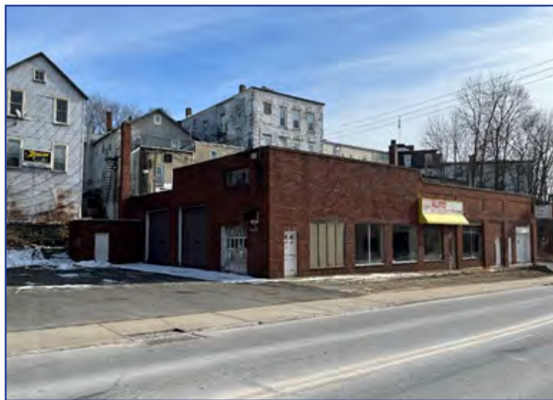
Image 105. North facing wall of former Capri Auto Body with the right of way connecting to Main Street behind the building
